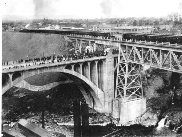
Spanning the bridge that spanned the falls. By 1912, the Union Pacific Railway bridge was constructed over the hydro station, the Monroe Street Bridge, and the falls, barely visible in the lower right corner. Note the extensive backfill placed to accommodate the rail grade. ( Eastern Washington State Historic Society )
