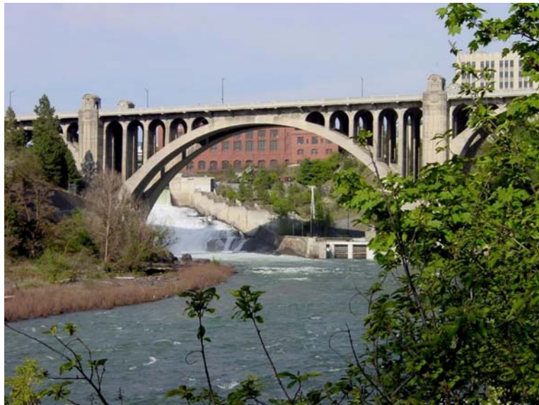
The Monroe Street Bridge, constructed in 1910, was the largest concrete-arch bridge in the world when built. It is currently scheduled to be reconstructed from the main arches up, and will allow the passage of the Centennial Trail beneath its northern landing. ( Friends of the Falls )
