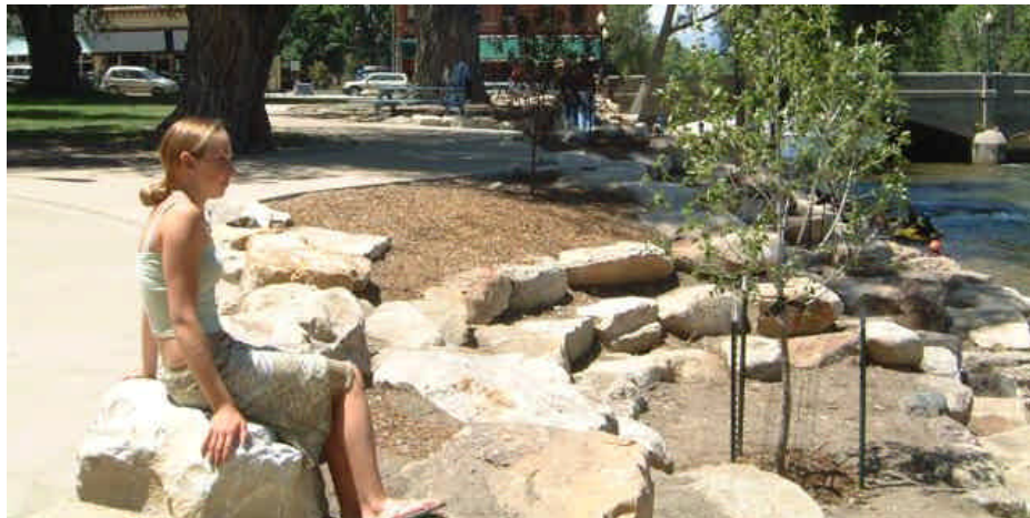
Figure 8. Bank terracing and planting terraces in Salida, Colorado
